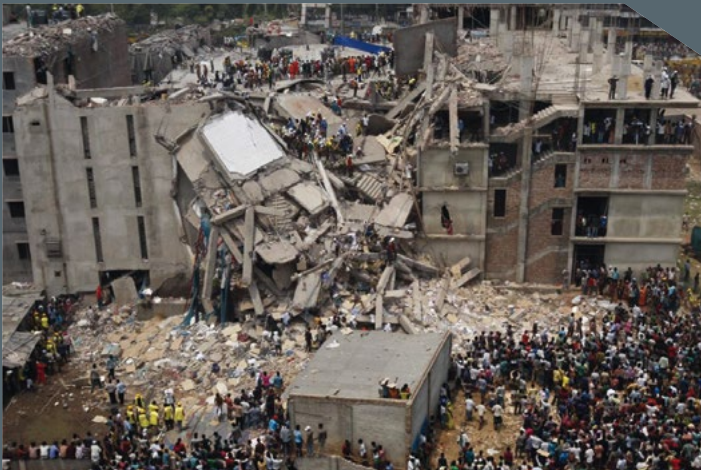
← The Rana Plaza factory building in Bangladesh after it collapsed in 2013.
